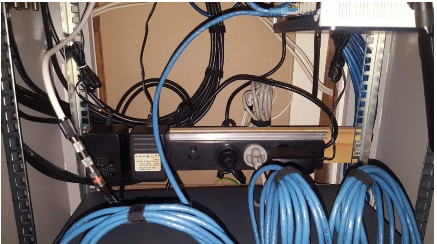
Photo 7: The new power board mounted on a piece of timber. Despite the wider spacing for plug packs on the right, due to the stupid design of one of them it still doesn't fit there and had to go on the far left.
