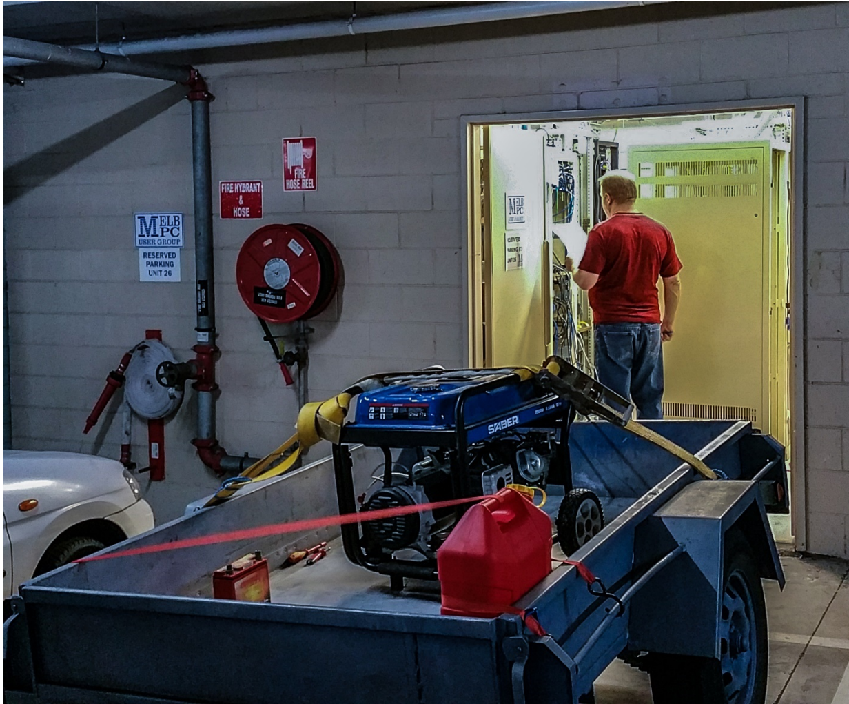
Generator connecting to the server room
