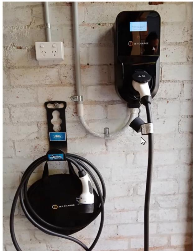
Figure 15 - Jet Charge Chargemate home charging station
