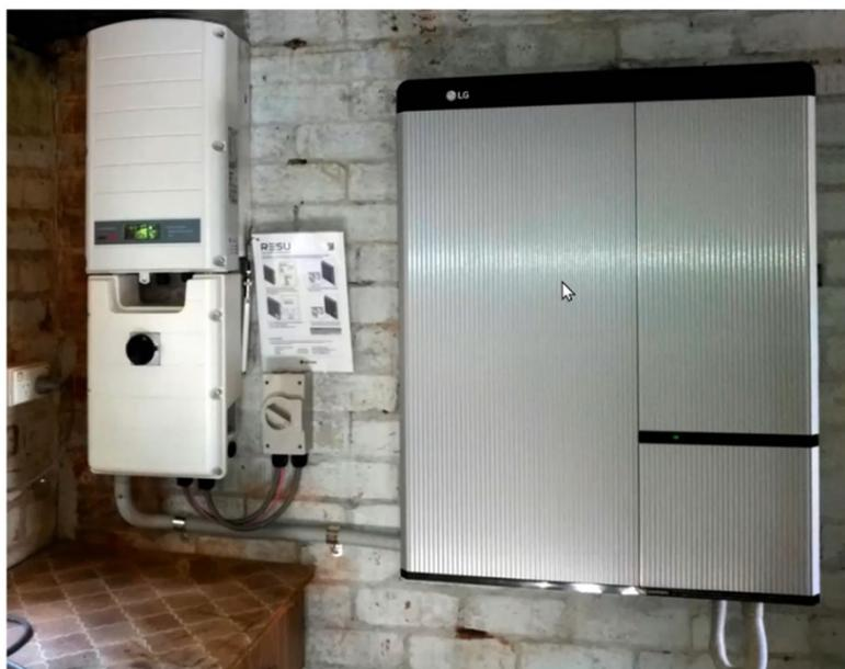
Figure 8 – Inverter & LG Battery installation
